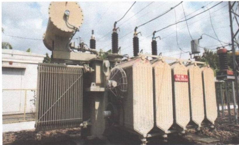
**Gambar 2.1 Transformator 3 Fasa**
